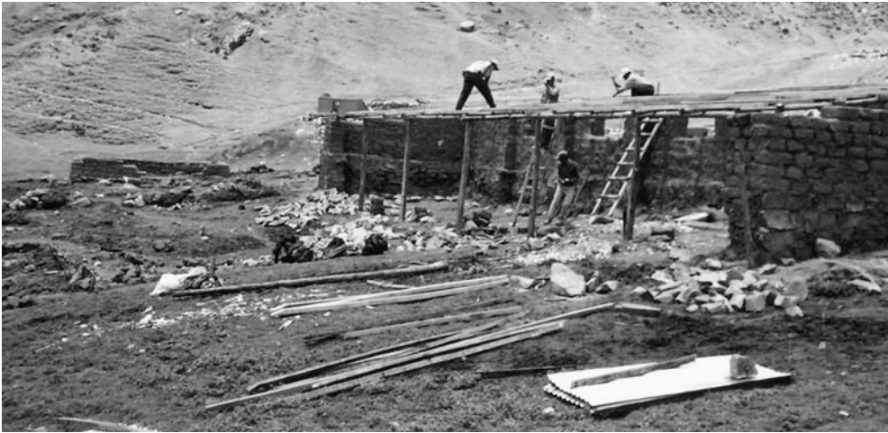
Construction of Alpaca shed: Photo: © Practical Action Peru
